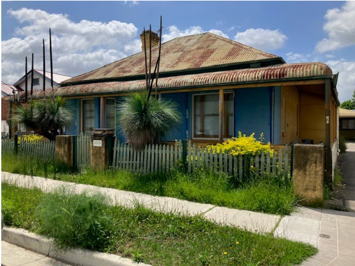
Figure 12 -Front (west) elevation of 158 Broomfield Street.
